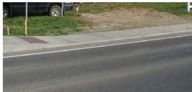
“Driveway” curb cut improperly replacing a wheelchair passing area in Oak Hill.
