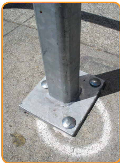
Figure 2-14: Flange concrete rack mounting (photo: Eric Anderson)
