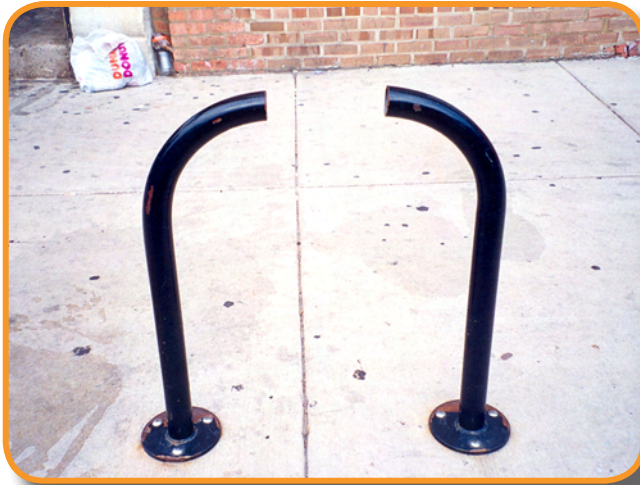
Figure 2-12: Cut round tubing rack (photo: Eric Anderson)
