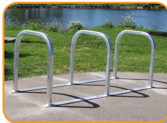
Figure 2-15: Rail mounted racks anchored to asphalt surface (photo: Heath Maddox)
