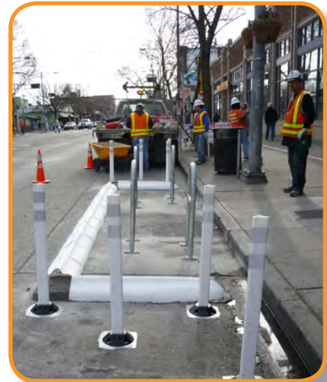
Figure 2-38: Concrete curbs are used to encourage entry from the sidewalk and protect bicycles (photo: City of Seattle, Wash.)
