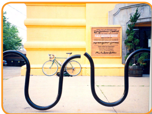
Figure 2-48: Round tubing bicycle racks are vulnerable to pipe cutters. (photo: Eric Anderson)
