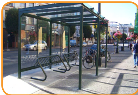
Figure 2-31: Victoria, B.C. placed a standard bus shelter on a curb extension (photo: John Luton, Capital Bike & Walk)
